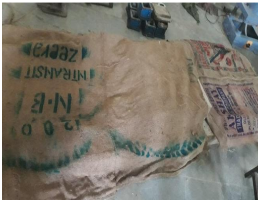
Fig.13. Curing of Casted Beams
